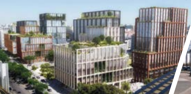
Entrecampos Complex, Lisbon (Portugal)
