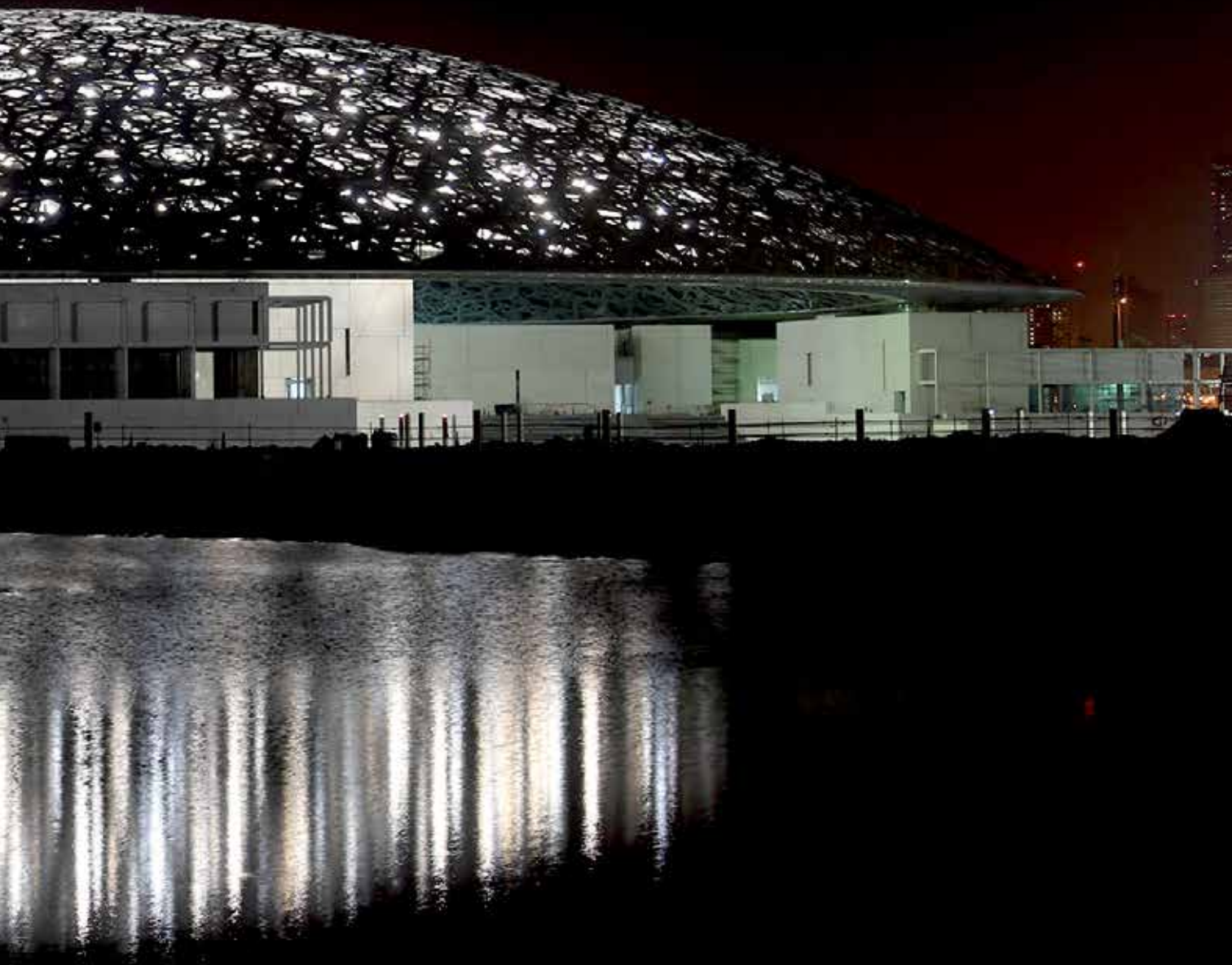
Louvre Abu Dhabi Museum (UAE) at the first lighting of the 4,500 steel tube lights of the dome
