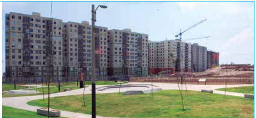
Condominium Parques de la Huaca, Lima (Peru). Engineering and project: GSJ Solutions / Execution: SANJOSE Constructora
