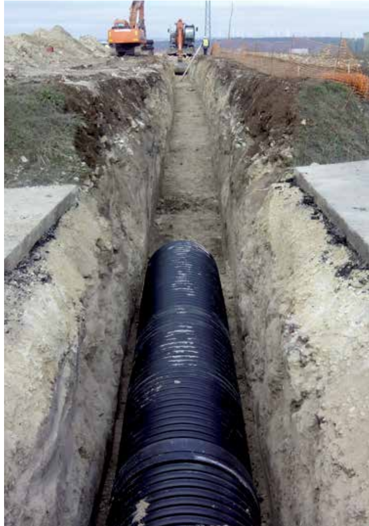
Drinkable water supply network and tank of Cortes, Burgos.
