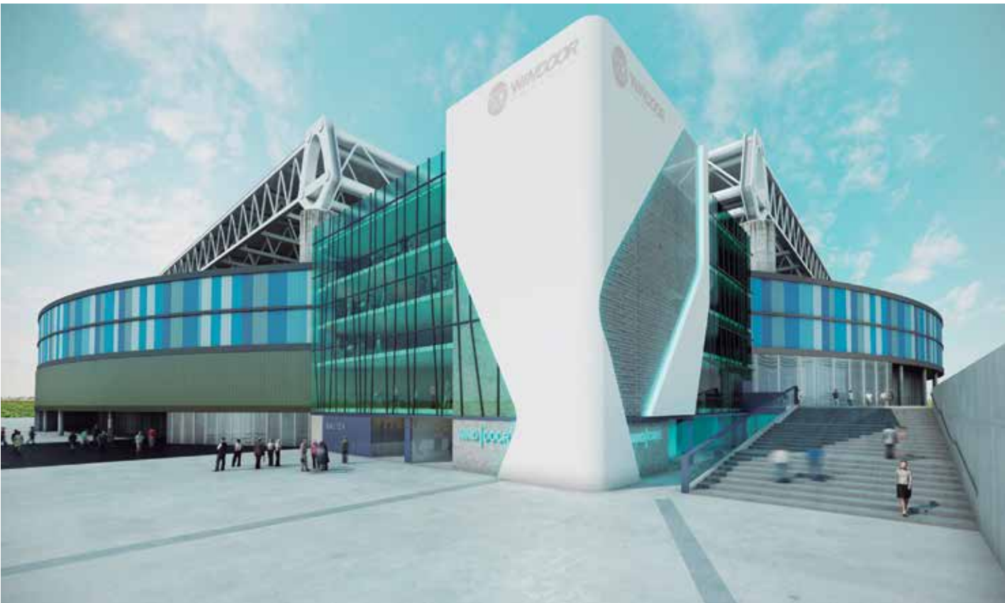
Wind Tunnel at the RCD Espanyol Stadium, Barcelona.
