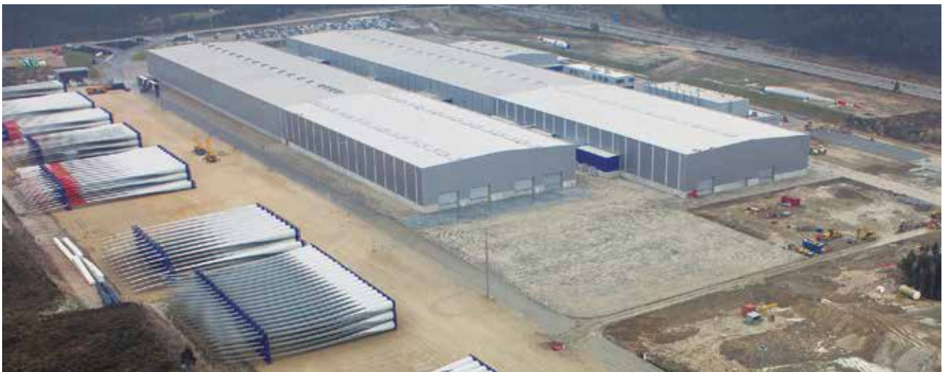
Enlargement of the factory of Ria Blades in Vagos, Aveiro (Portugal).
