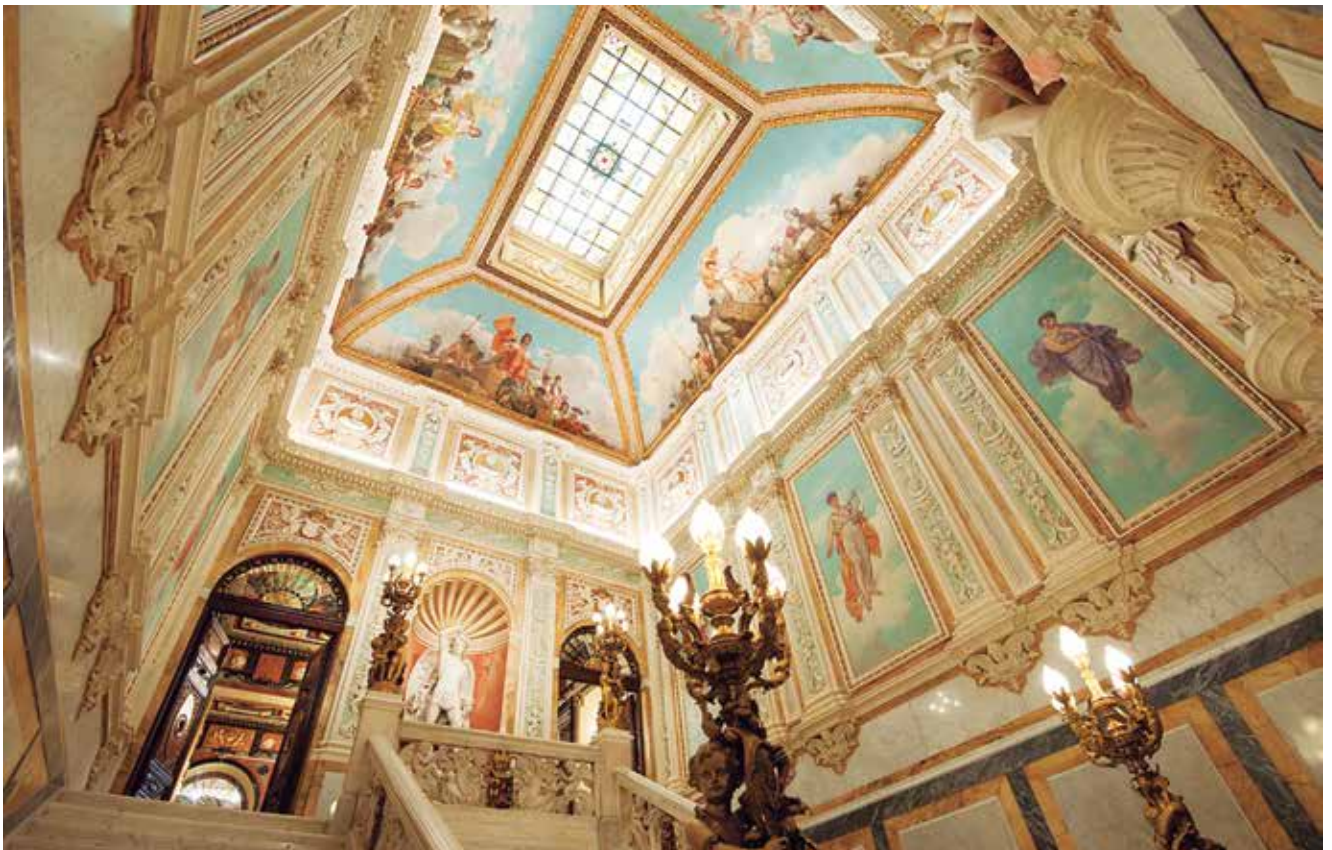
Refurbishment of the Santoña Palace of Madrid
