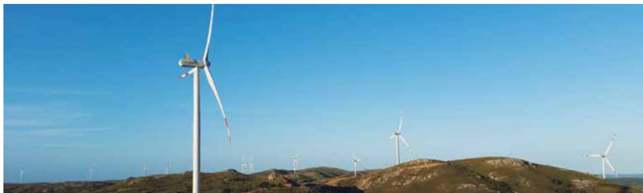
Wind farms in Uruguay (90MW). Engineering and project GSJ Solutions / Execution SANJOSE Constructora
