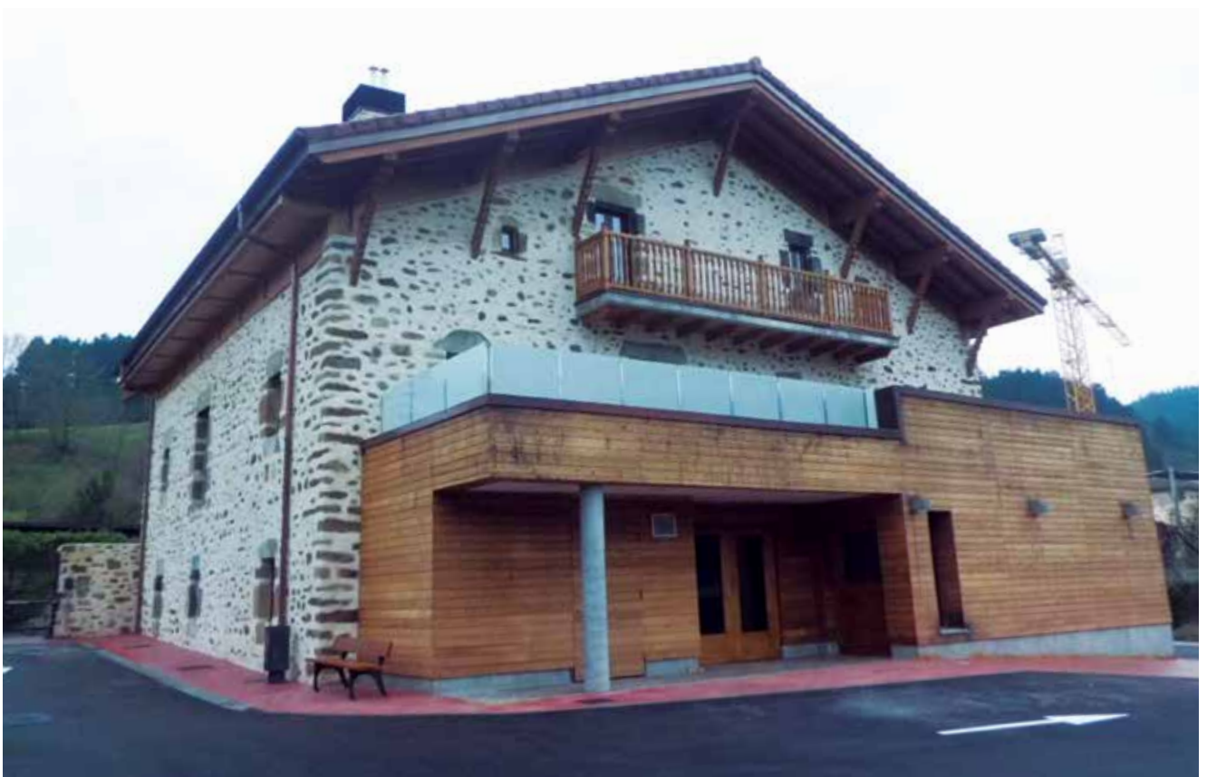
Rehabilitation of the multi-purpose building of Luyando, Alava.
