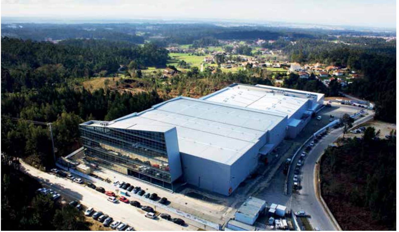
Enlargement of the factory of Aspock Logistics in Vila de Cucujães, Oliveira de Azemeis (Portugal)
