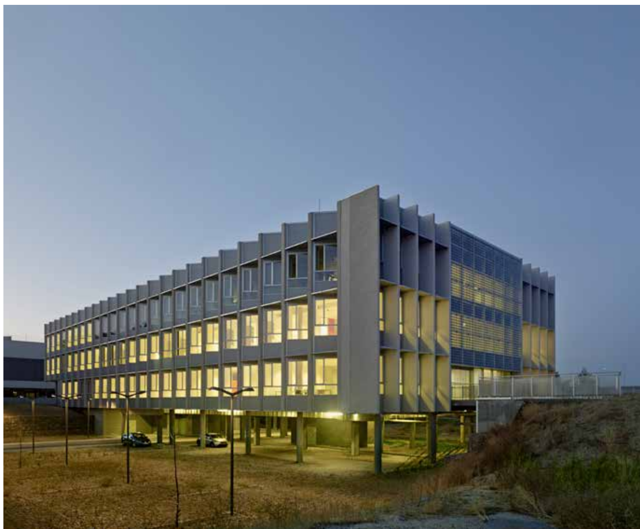
LUCIA Building, University of Valladolid (Spain). Certified with 98 points by Leed Platinum as Europe's most sustainable building and the second worldwide
