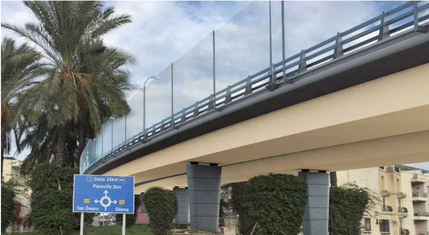
Flyover at EA15 In Kappara, Malta. Engineering and project: GSJ Solutions / Execution: SANJOSE Constructora
