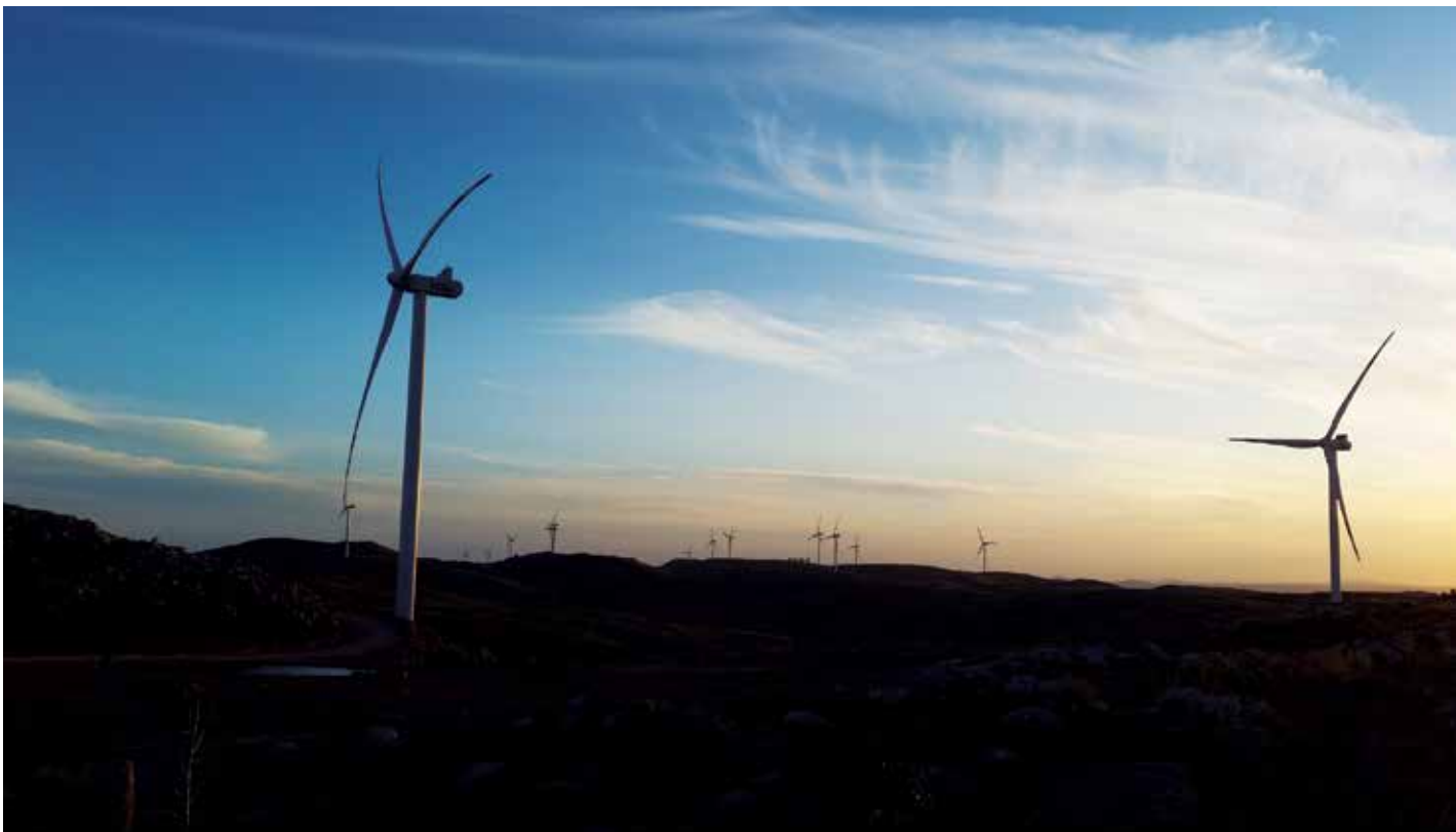
Wind farms in Uruguay (90MW) Engineering and project: GSJ Solutions / Execution: SANJOSE Constructora
