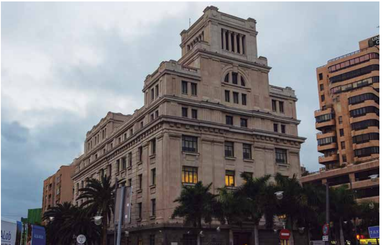
Refurbishment of the Main Office of Correos y Telegrafos of Las Palmas de Gran Canaria.
