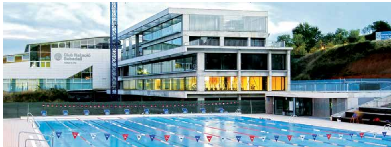
Enlargement of the Swimming Club of Sabadell, Barcelona (Spain)
