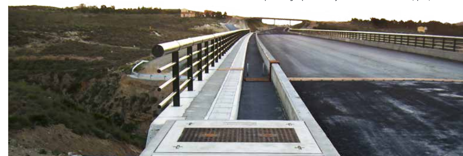
Stretch Vera - Los Gallardos. Spanish High Speed Railway Line AVE Almeria - Murcia (Spain)
