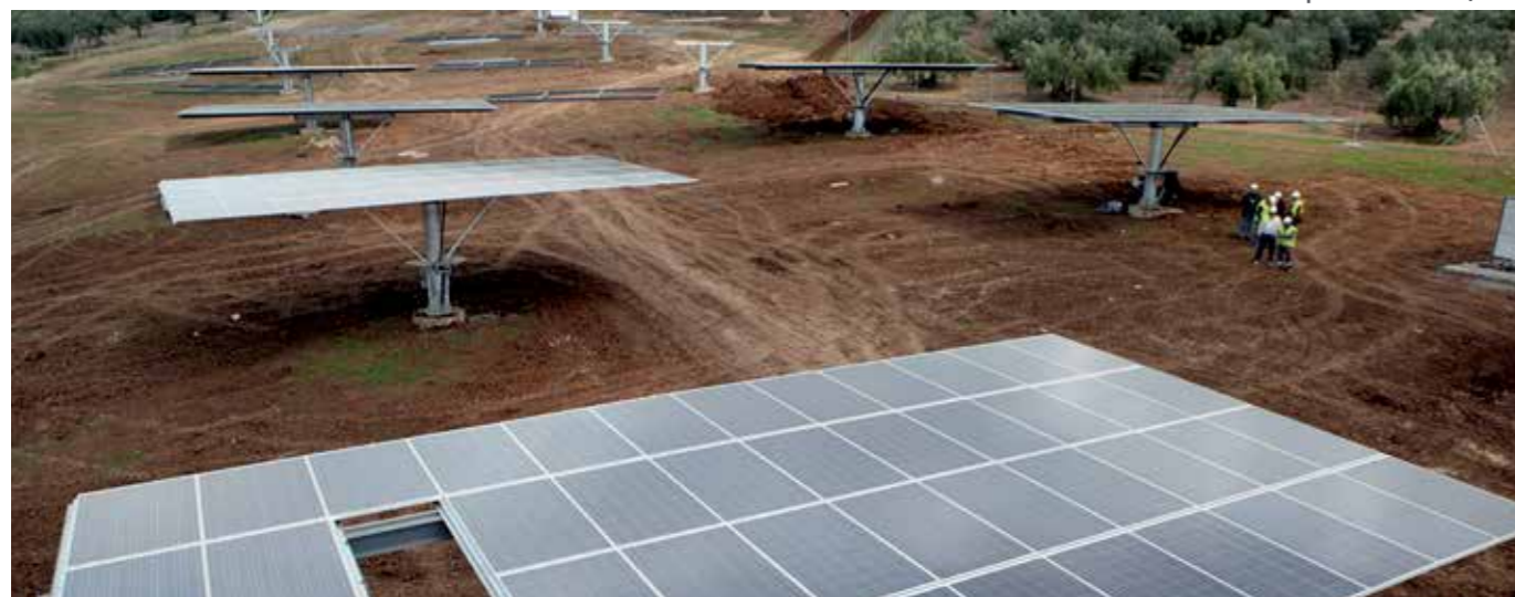
5.4 MW solar plant in Alcaudete, Jaen
