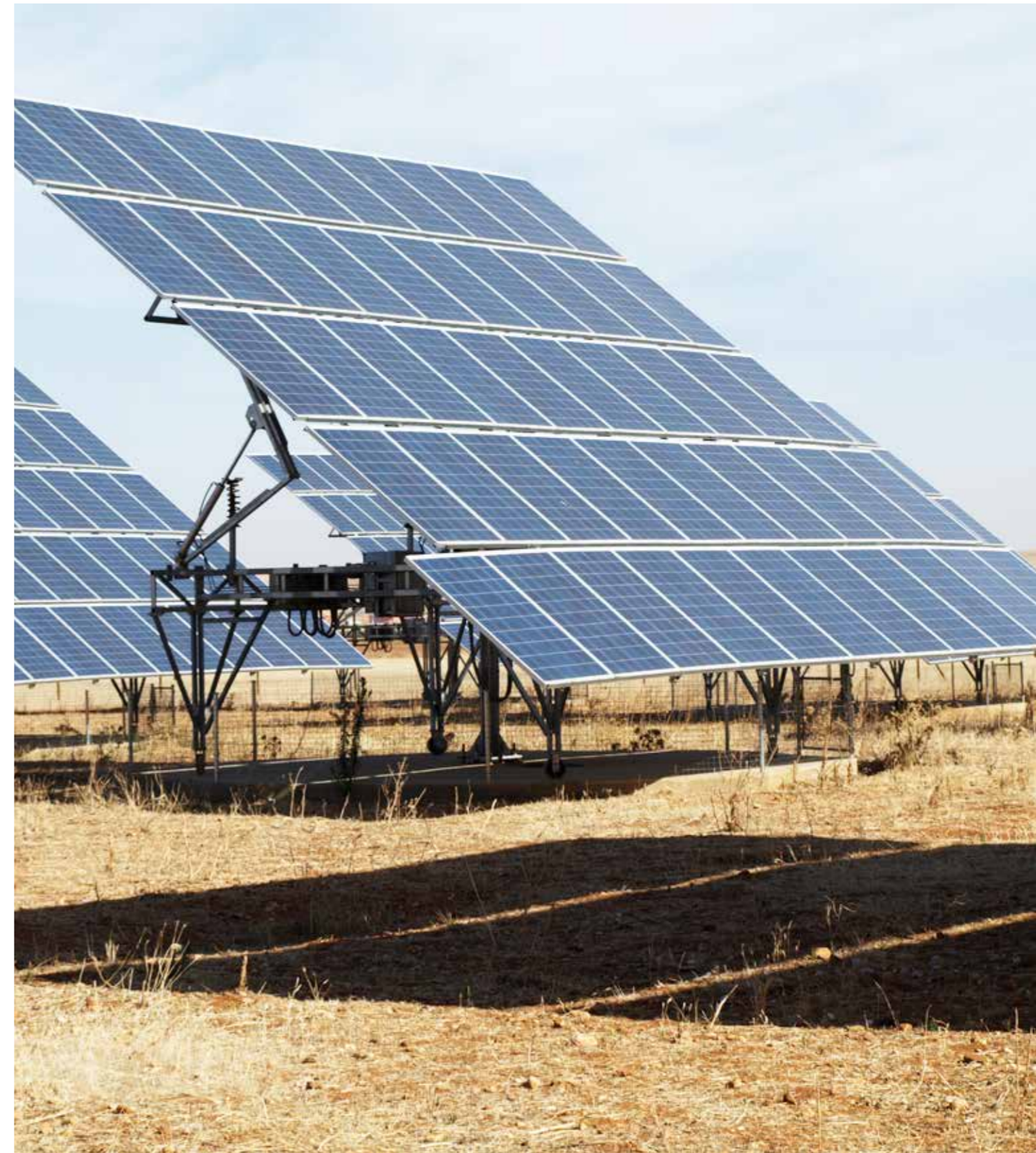
3.33 MW solar plant in Toro, Zamora
