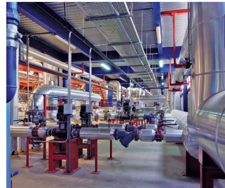
DHC pumping system
