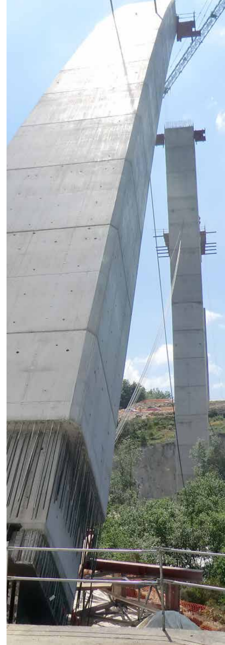
Arnoia Viaduct, stretch Miaman - Ponte Ambía (Orense). High Speed Railway Madrid-Galicia (Spain)
