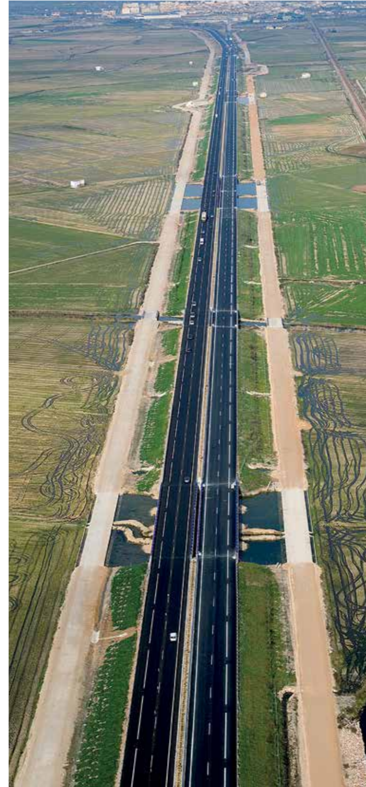
STRETCH SUECA - SOLLANA. DOUBLING OF NATIONAL ROAD N-332, ALMERIA - VALENCIA
